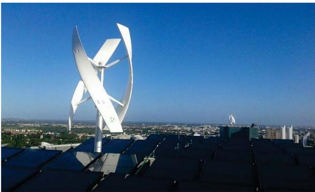
**FIGURE 2.10:** Building Integrated Microturbine
